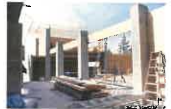
Construction of Ochoco Addition (1981)
