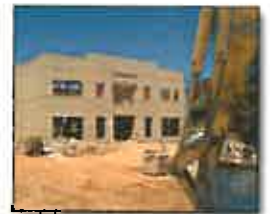
The Library under construction.
