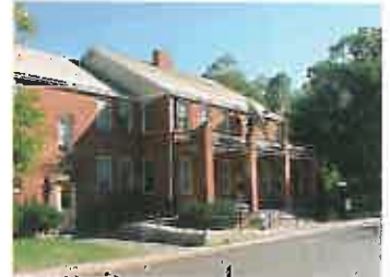
Building housing the Warm Springs College Center.
