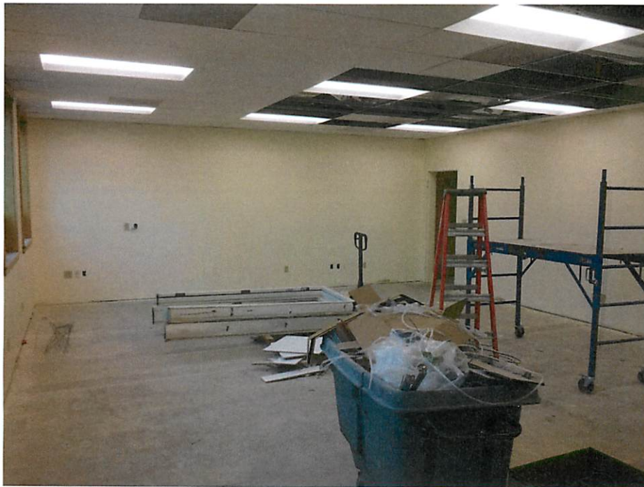
Data, Lights & Paint – Classroom 128, Redmond Building One
