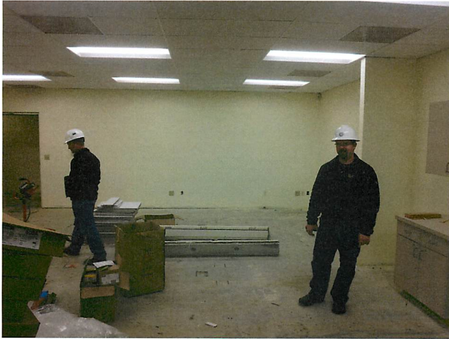
Data, Lights & Paint – Classroom 122, Redmond Building One
