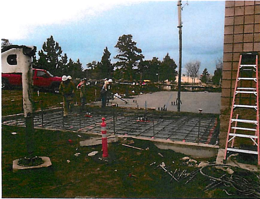
Placing Slab on Grade
