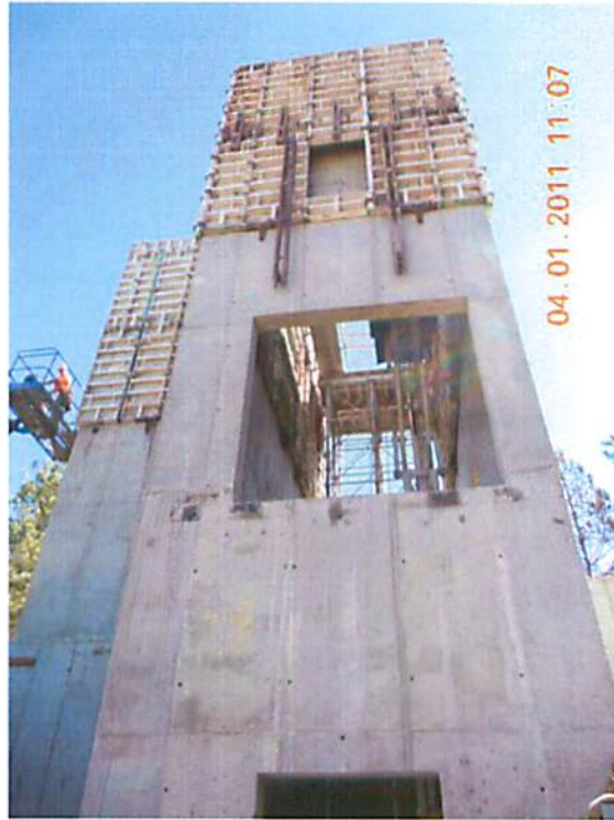
Last lift of the east tower formwork.
