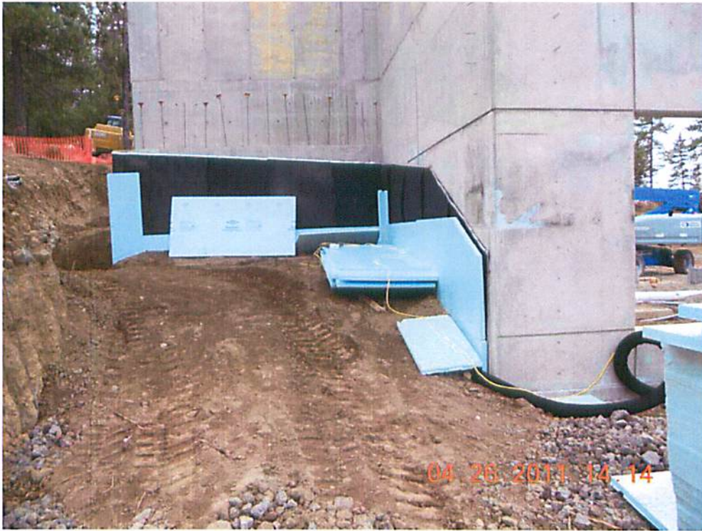
Waterproofing, insulation, footing drain, and backfill at east walls.
