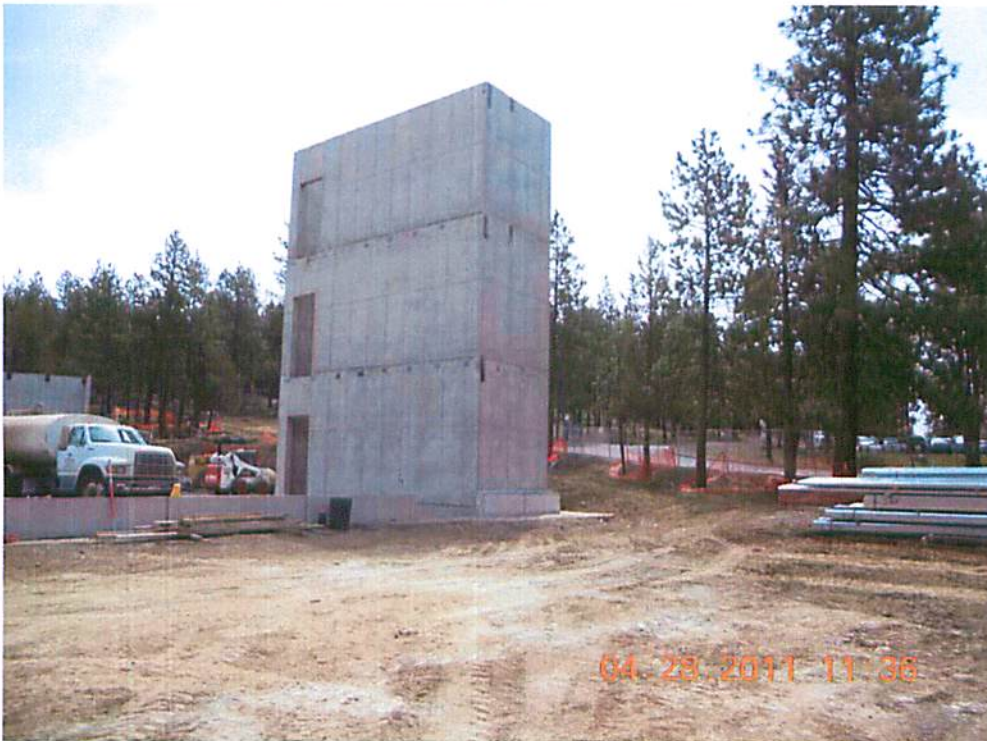
West stair tower complete and ready for structural steel.
