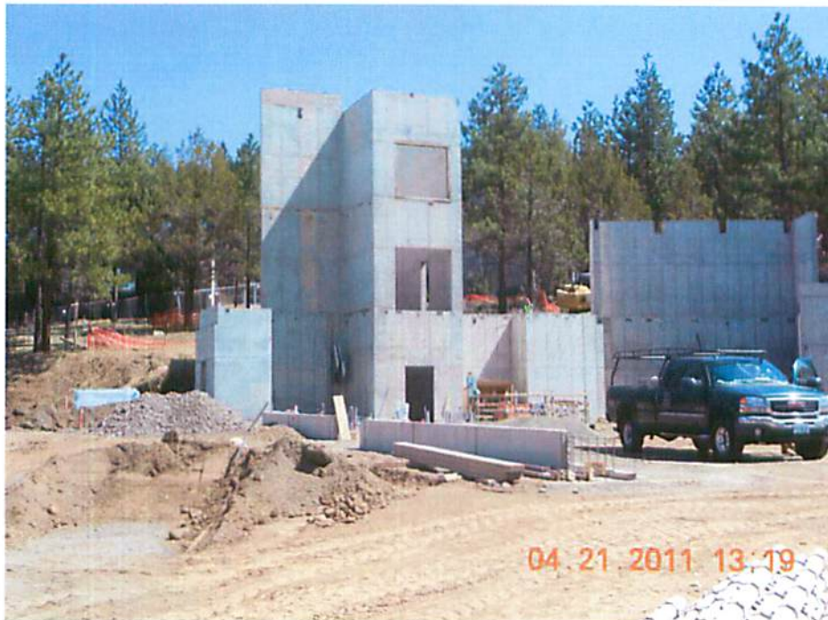
East walls ready for structural steel
