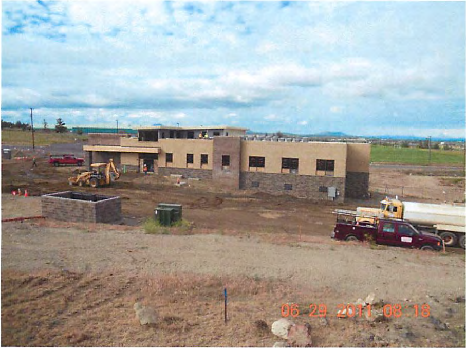
Exterior Nearly Complete.
