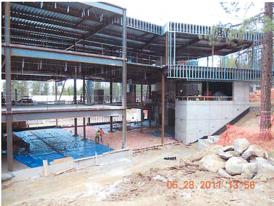
Slab on Grade Prep. And Exterior Stud Framing
