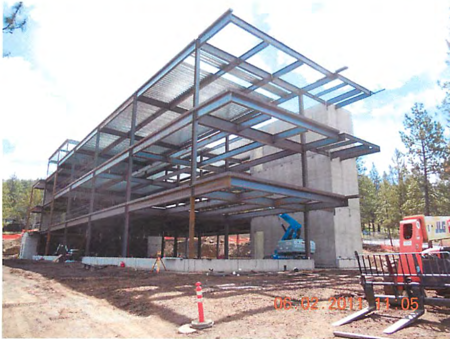
Steel Erection Nearly Complete
