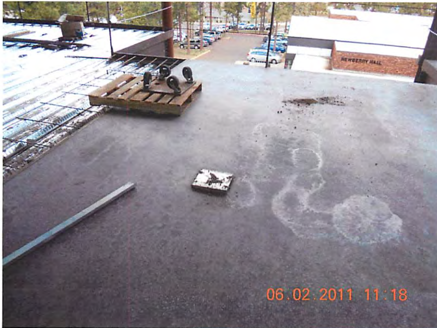
Roof Slab 30% Complete
