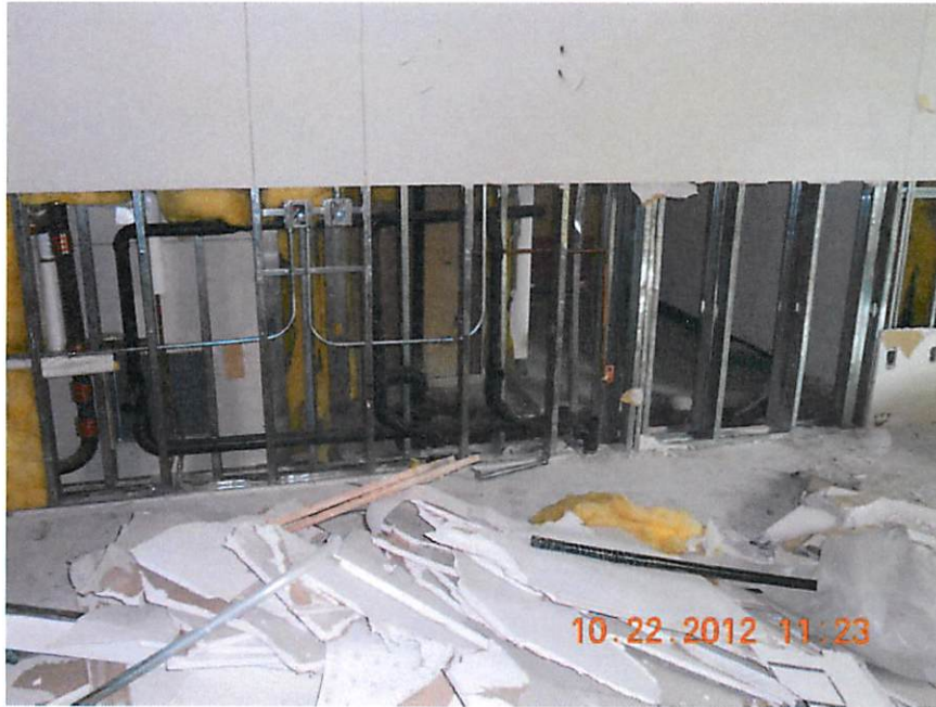
Plumbing Changes in Remodeled General Science Classroom
