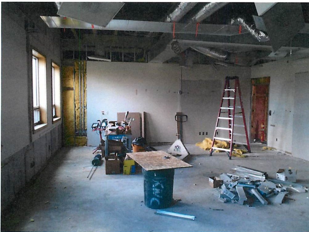
Demolition – Classroom 128, Redmond Building One
