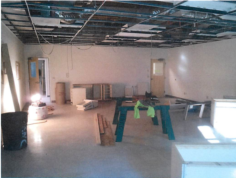
Demolition – Classroom 122, Redmond Building One
