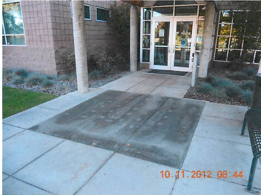
Front Entrance ADA upgrades
