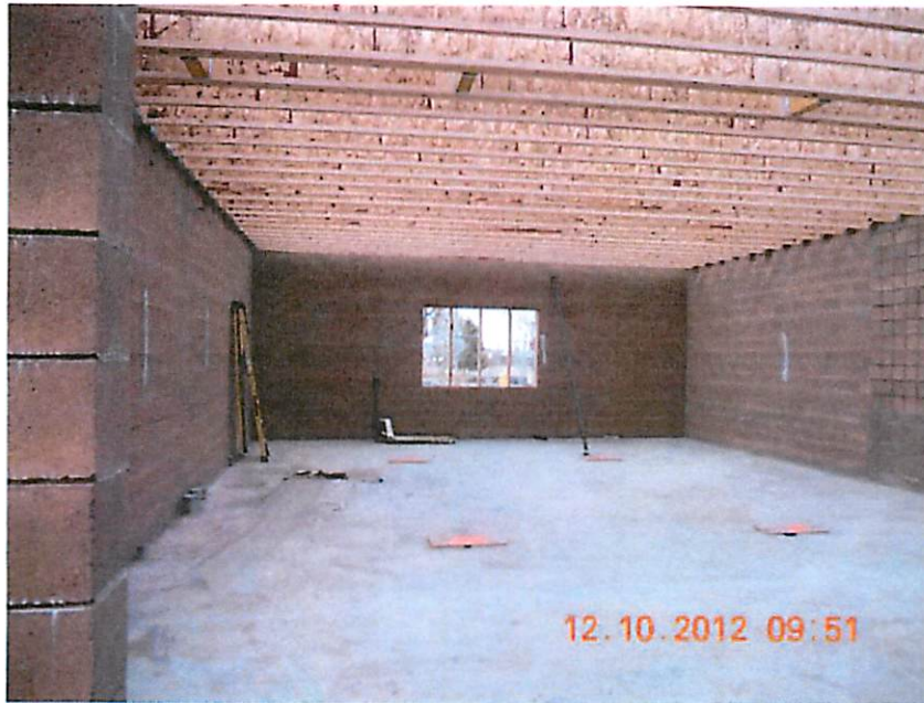
Roof Joists in Place on Addition
