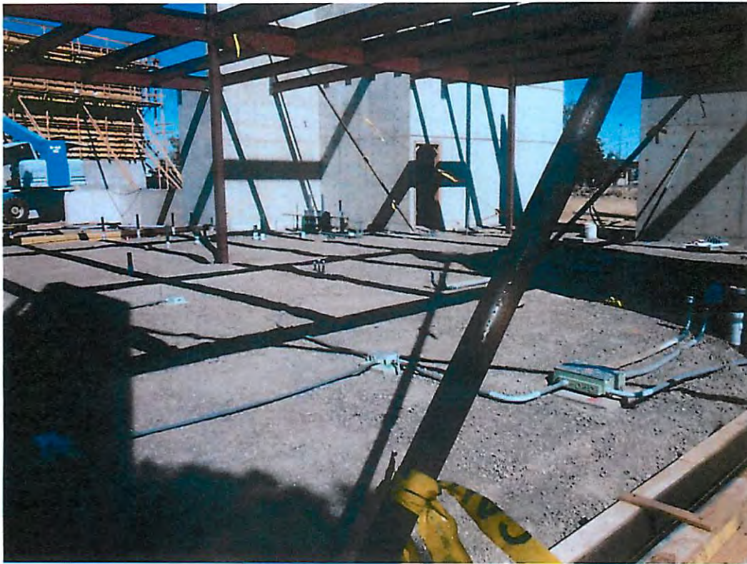
Floorbox and Conduit Installation – South wing, Redmond Technology Center
