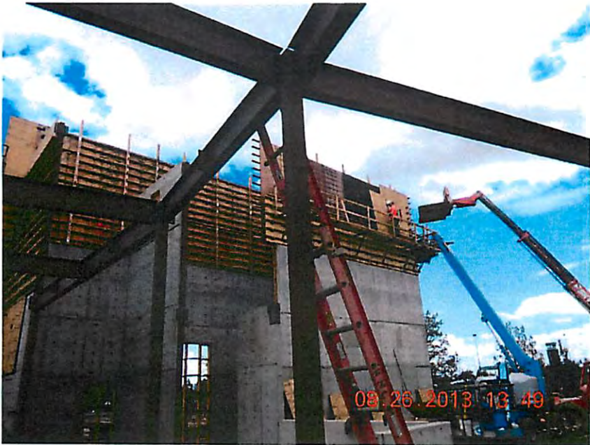
Steel and Concrete at Core Classrooms
