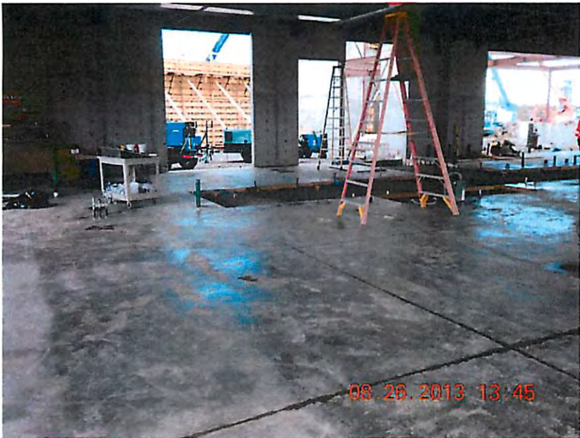
Slab on Grade at South Wing
