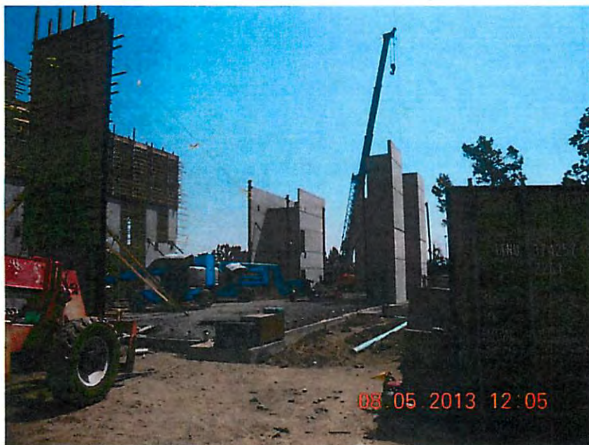
Structural Steel Starts at South Wing
