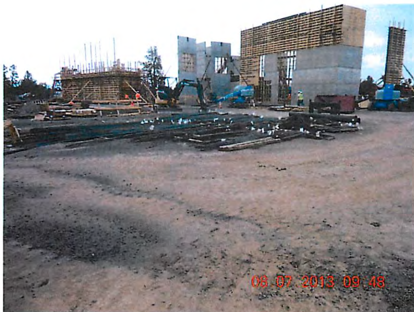
Concrete Walls Continue
