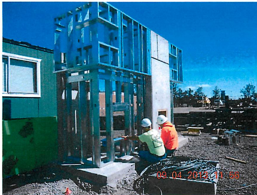
Exterior Enclosure Mock-up
