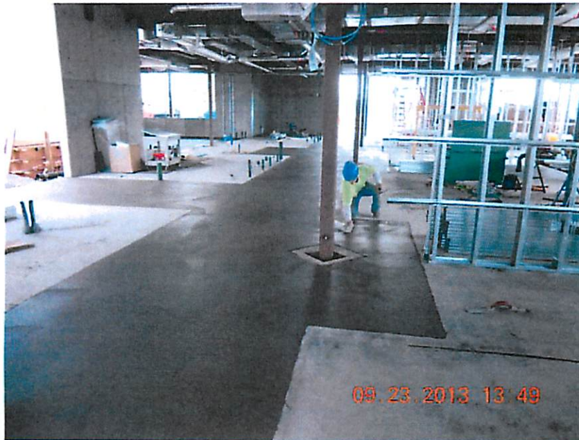
Polished Concrete Slab on Grade Placement
