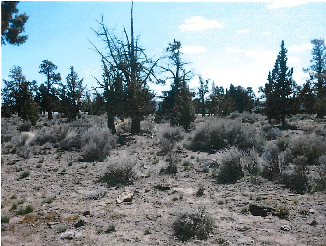
Construction Site from Vault – Redmond Technology Center
