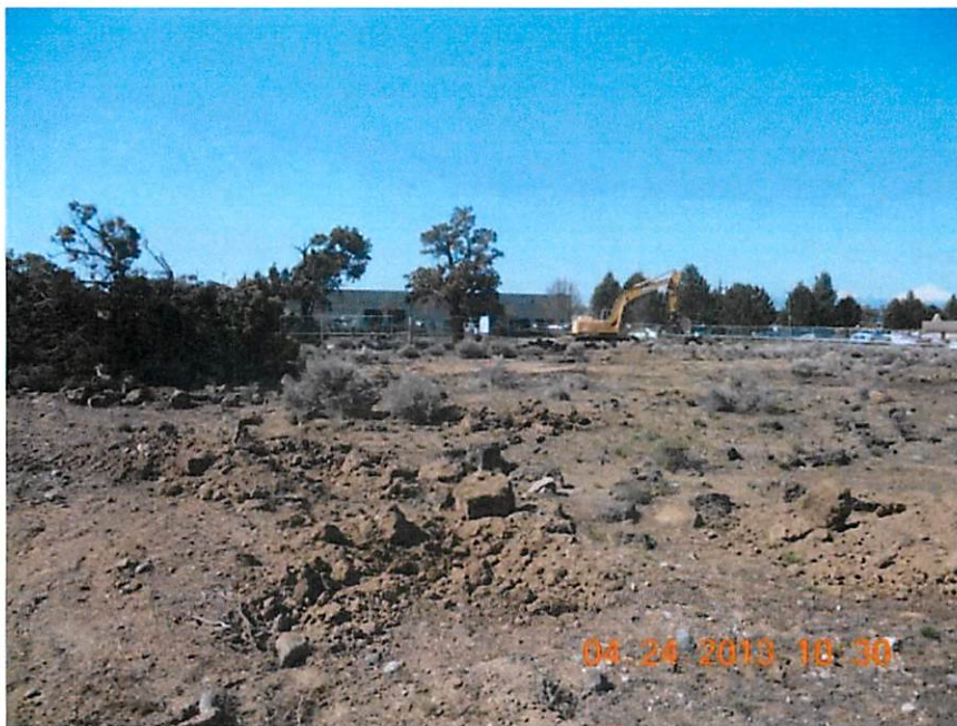
Clearing the Site
