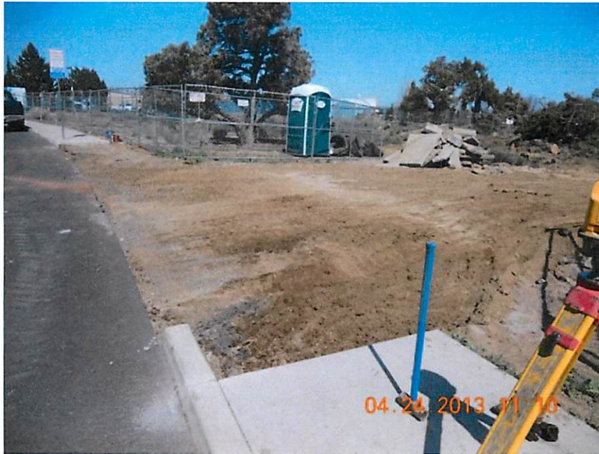
Construction Entrance off of Salmon Dr.
