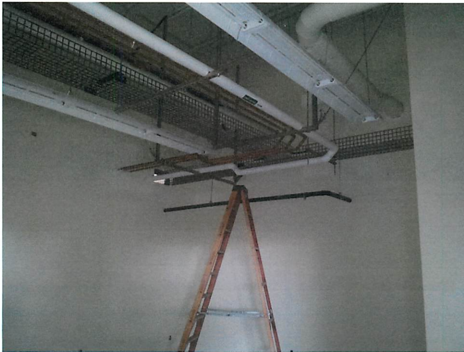
Cable Tray Installation – Resource Room 112
