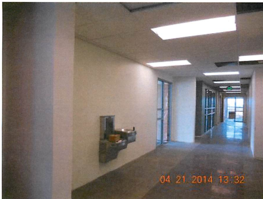
Lower Floor Hallway on South Side
