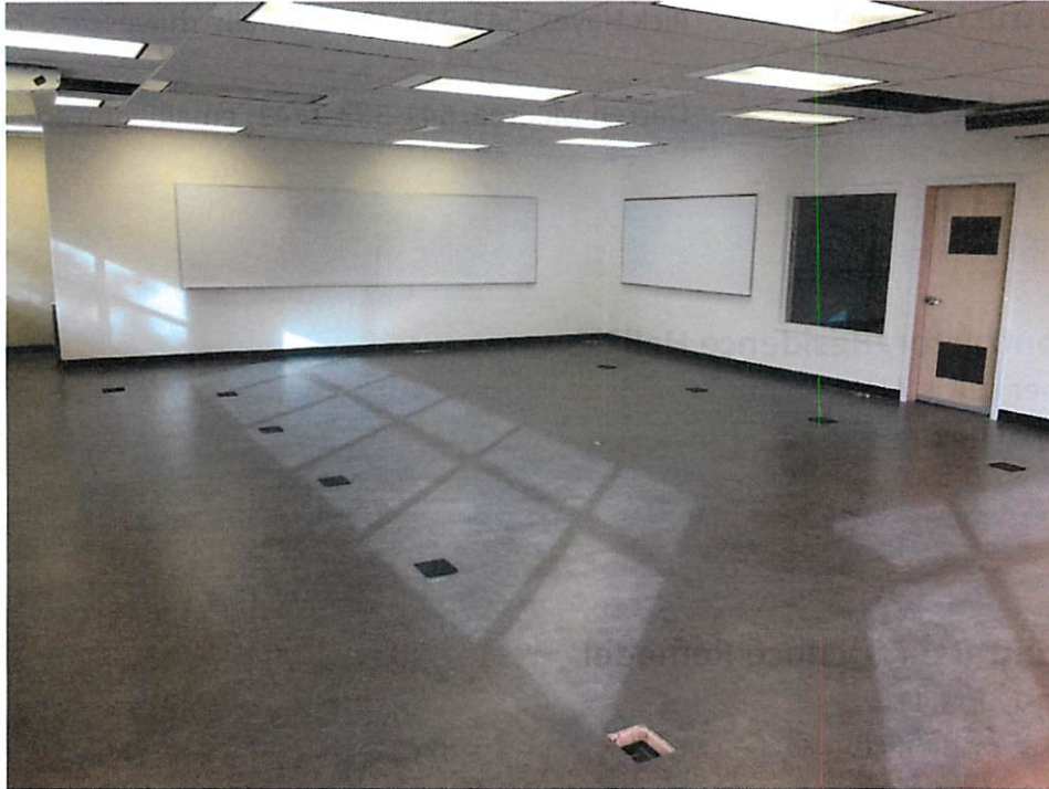
Computer Classroom Floorbox Install – Pioneer 232 Remodel
