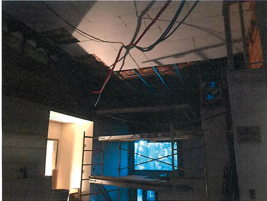
Upgrading the Fire Rating
