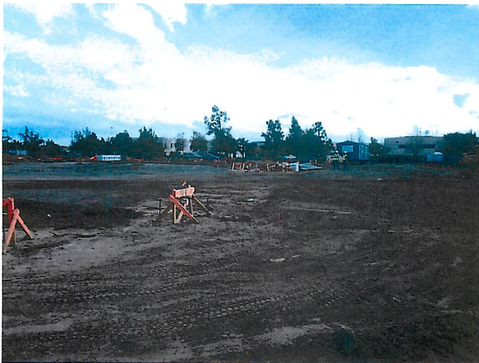
Construction Site from Vault – Redmond Technology Center
