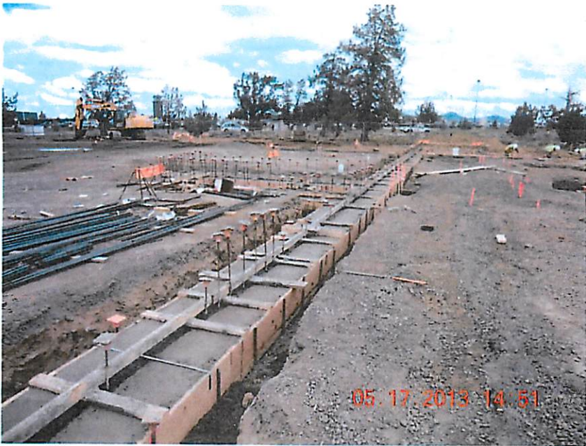
South Footings Placed
