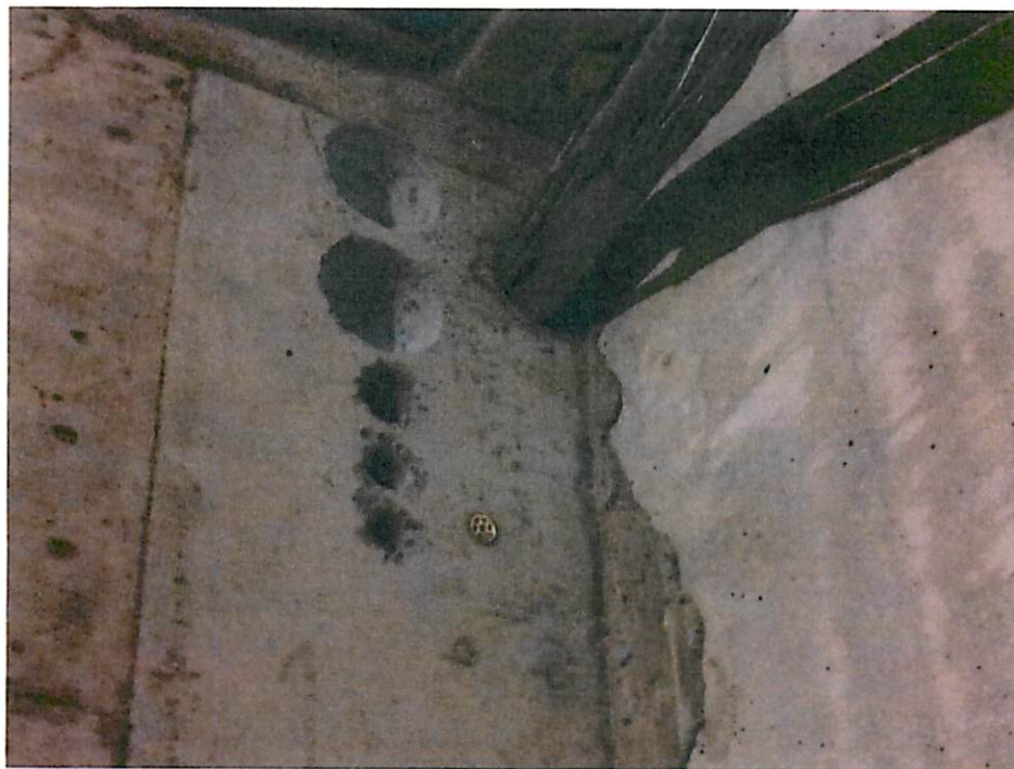
Core drillings for future low-voltage chases – MDF, Grandview
