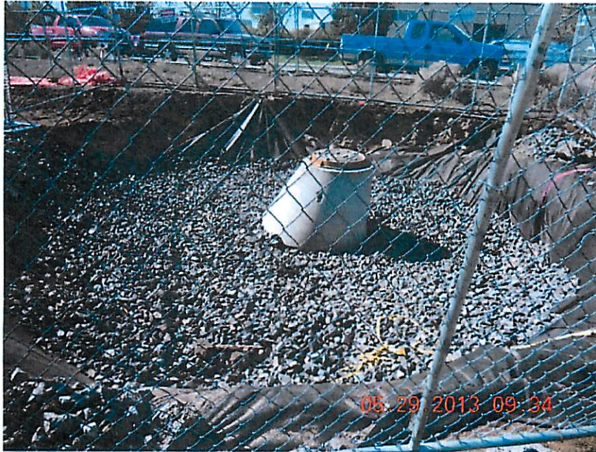
Drywell Installed
