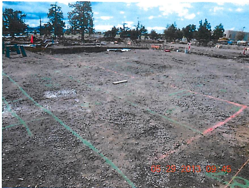
Final Portion of Footings Marked for Excavation
