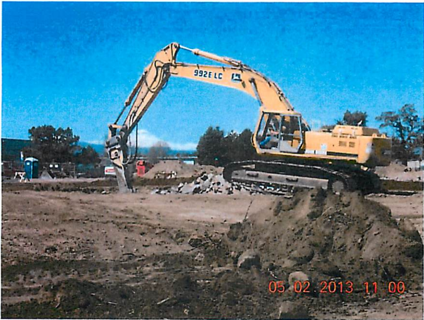
Elevator Pit Excavation
