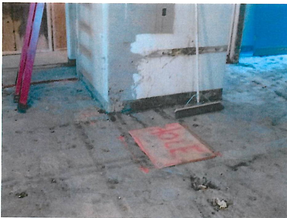
Future low-voltage chase construction – Office Area, Grandview
