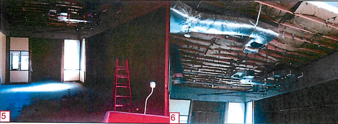
5 Bathrooms demolished and ready for framing. 6 Roof structure of bathrooms
