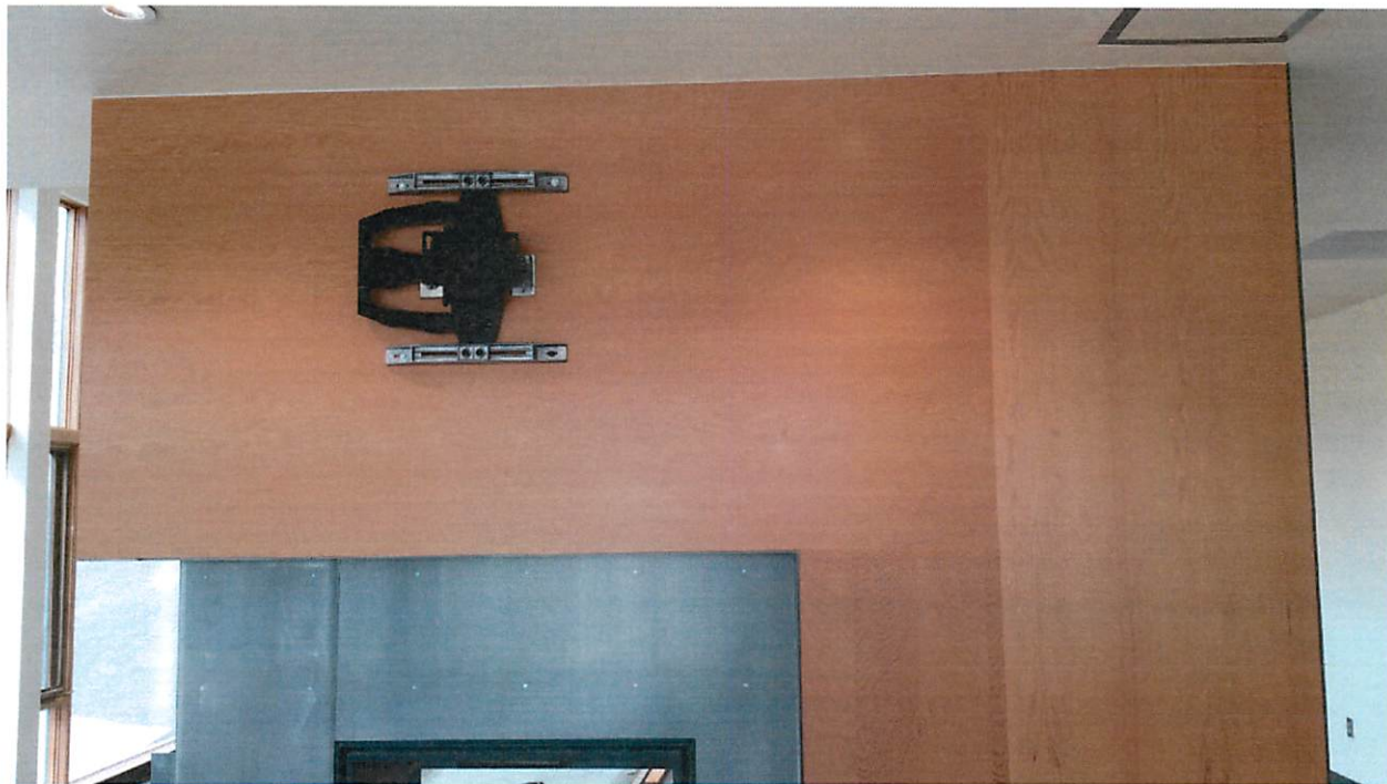
Television Installation – Residence Hall, Lounge Area
