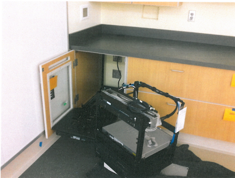
Installation of A/V Equipment Rack in Casework – Health Careers, Nursing
