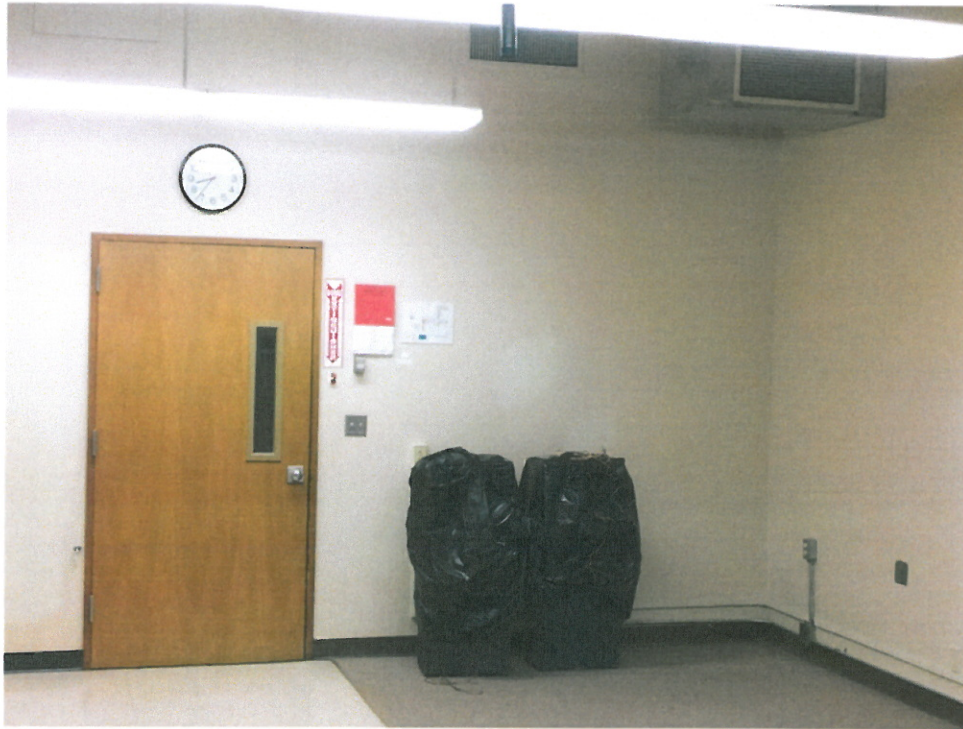
Computer Lab – Chandler Building, Room 207 (Before)
