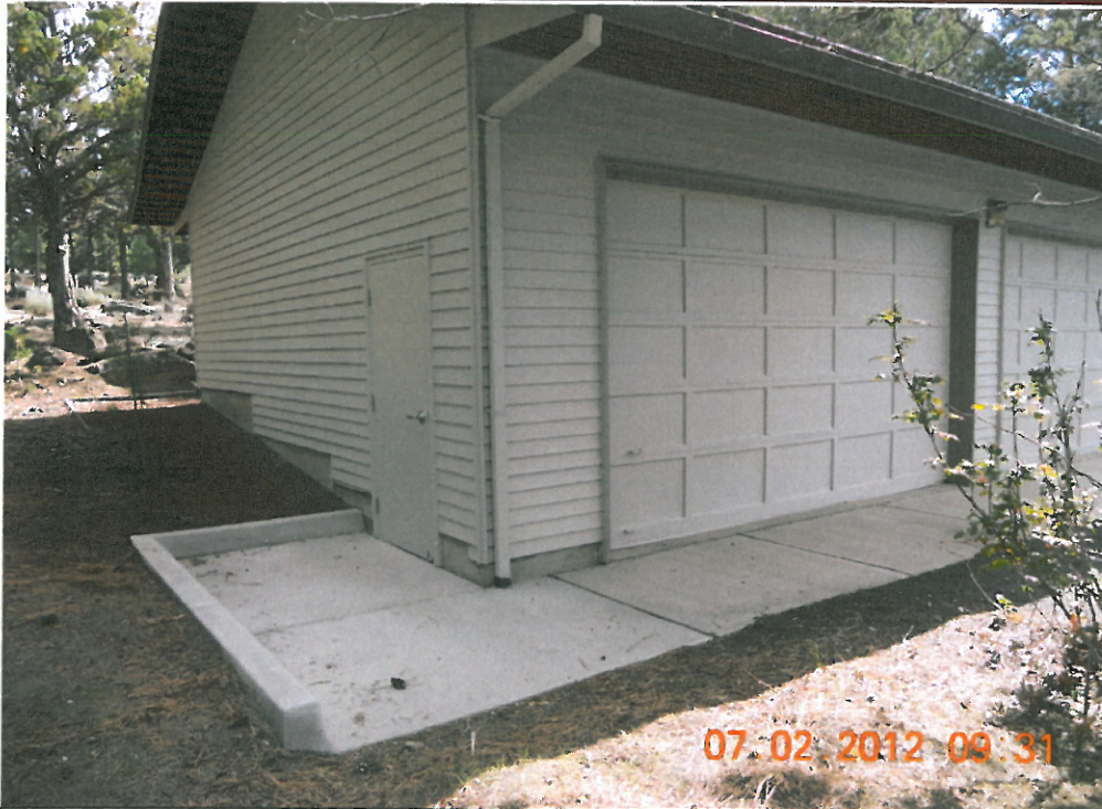
Garage division and exterior door installation complete. Exterior painting complete.
