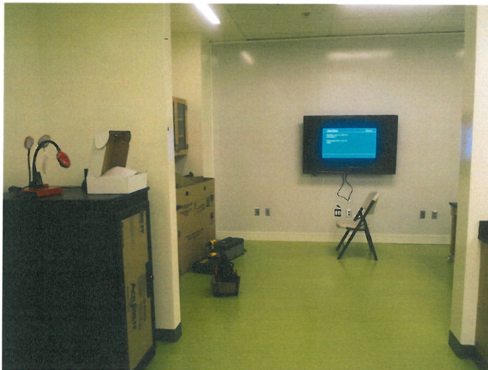
Installation of AV Rack and LCD Panel – Science Building, Lab 120
