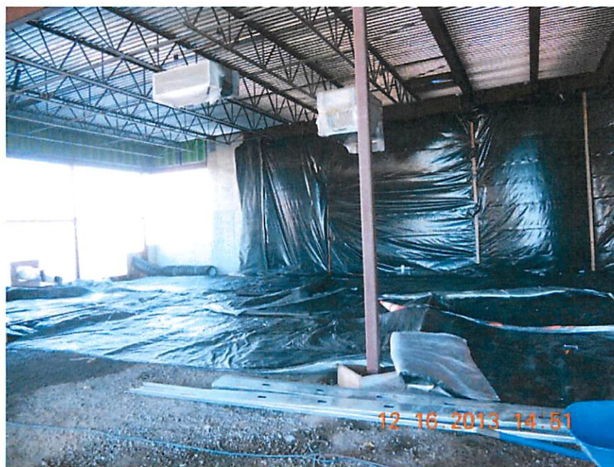
North Wing – Temporary warming measures
