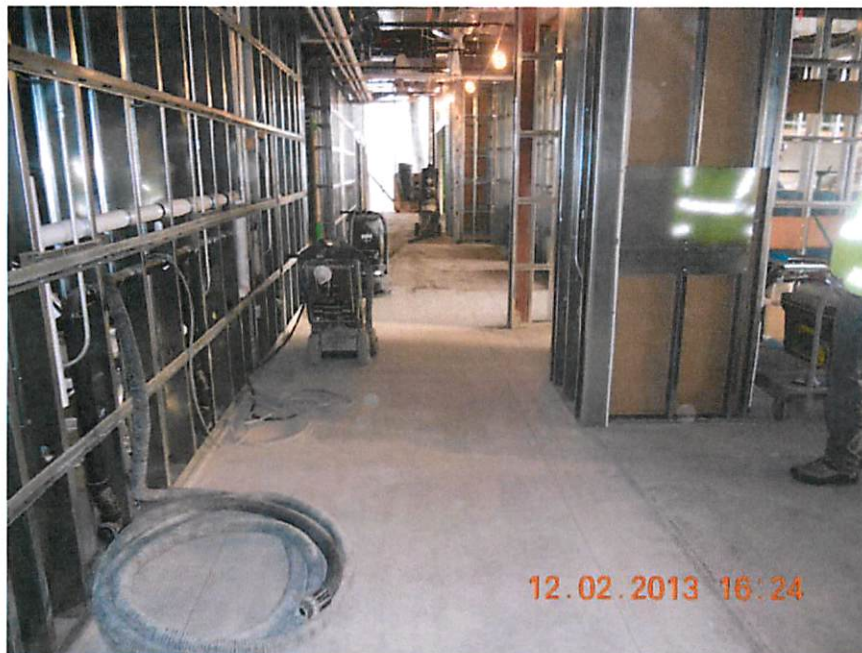
Polished Concrete grinding
