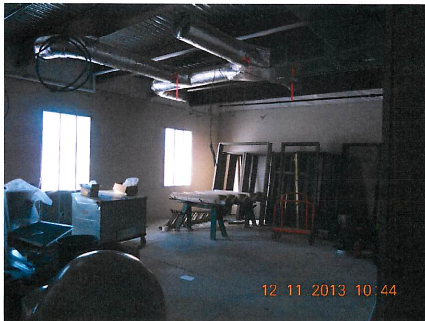
South Wing – General Purpose Classroom
