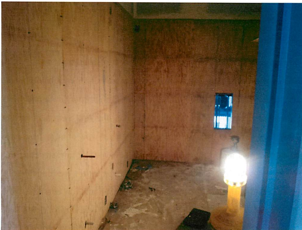
Fire-Treated Backing – MDF, 2 nd Floor
