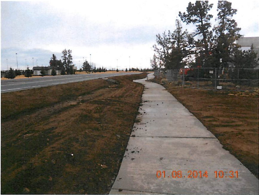
Airport way Sidewalk and Grading
