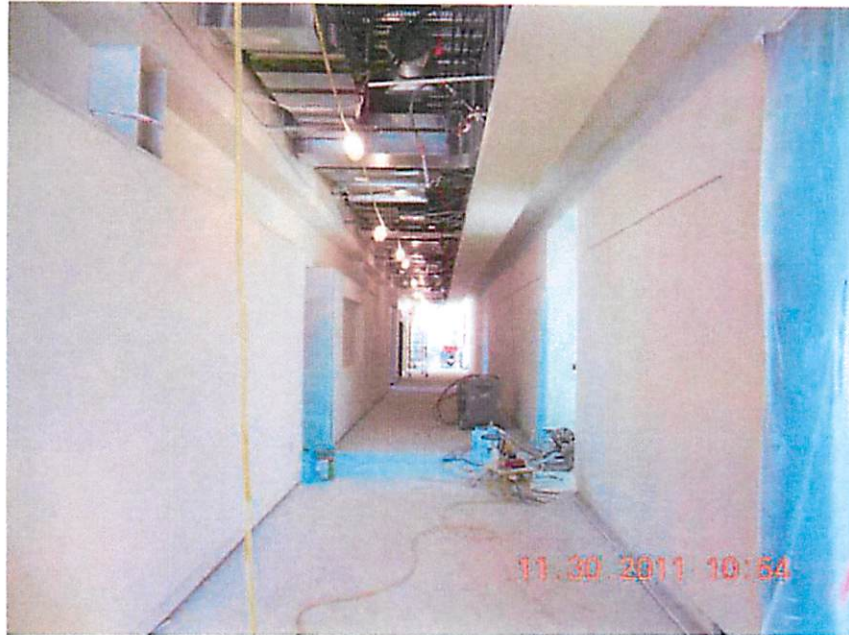
2 nd Floor Hall Ready for Paint
