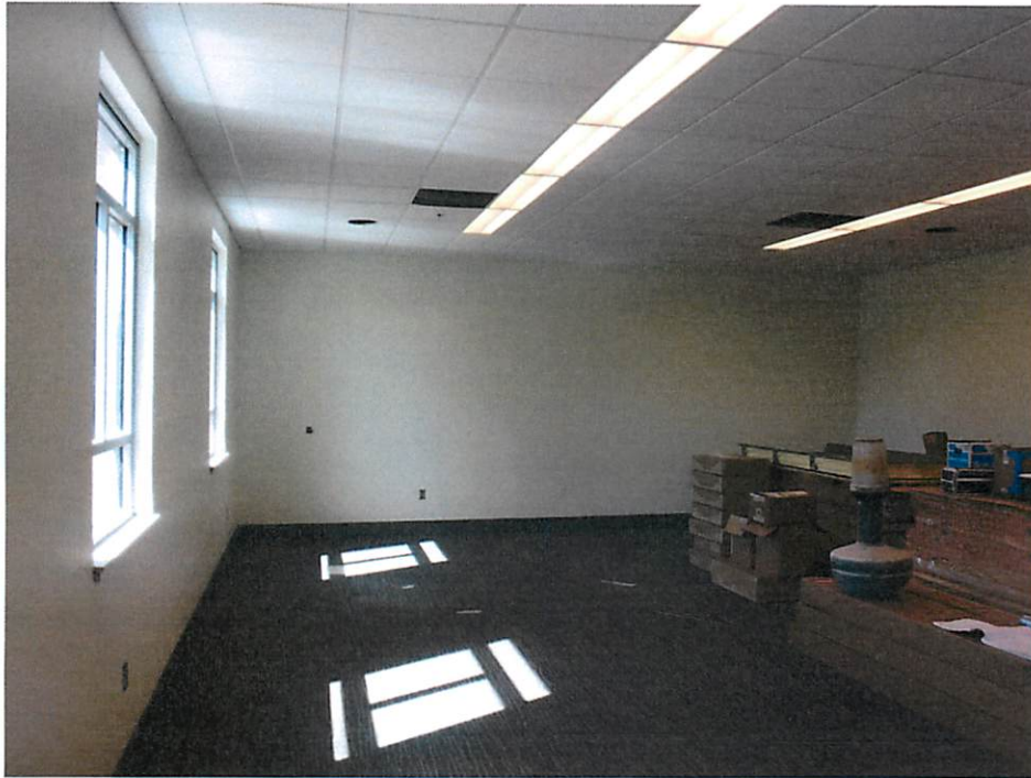
Projection Wall & Speaker Tiles – Classroom 134
