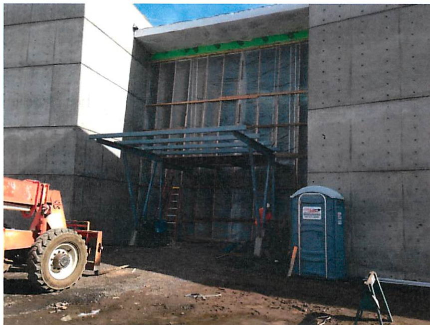
Main Entrance Canopy
