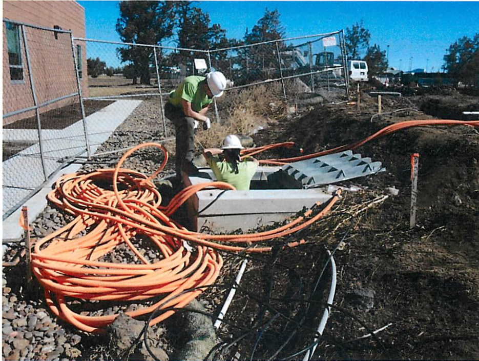
Copper & Fiber Innerduct Installation – Communications Vault
