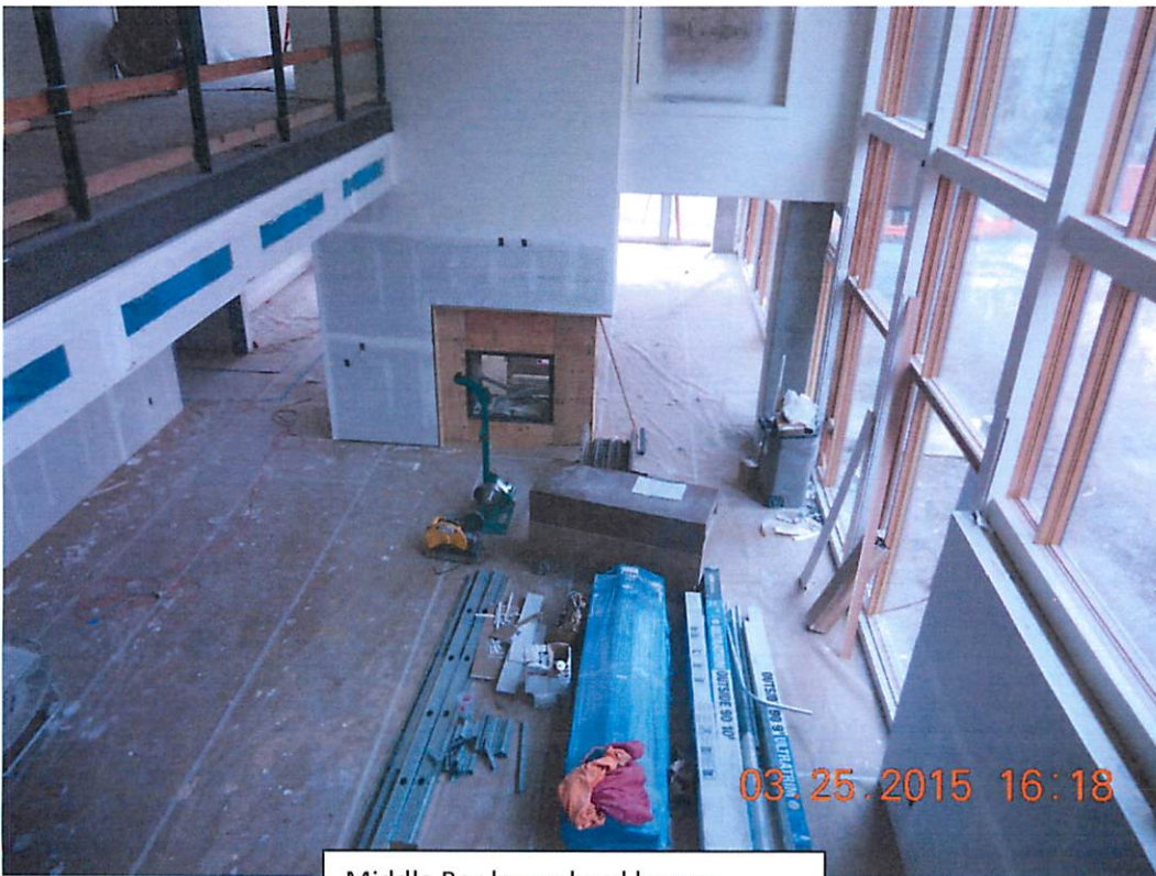
Middle Bar lower level lounge
