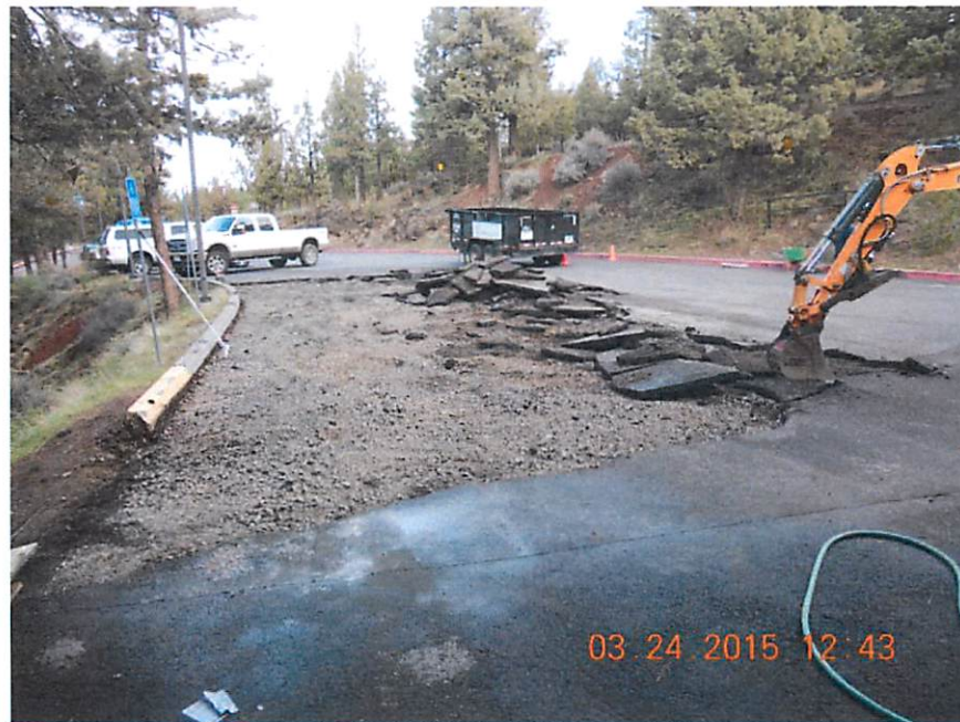
ADA Parking Improvement
