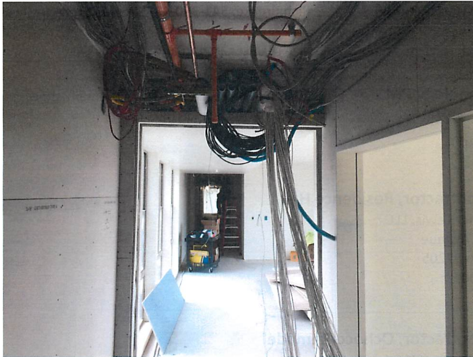
CAT6 Network Cable Installation in Progress – Lower Bar, Residence Hall
