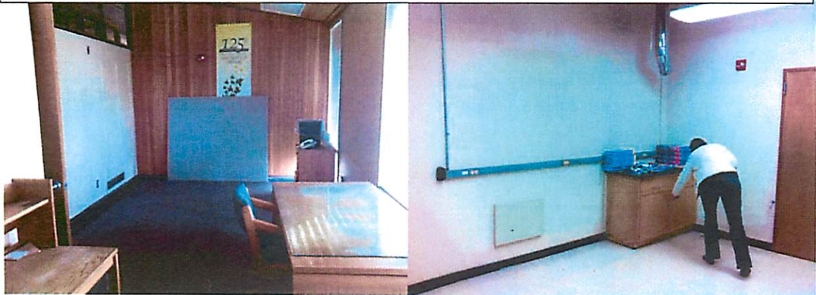
Office admin area to be expanded for 5 stations. Classroom to be converted to computer lab.
