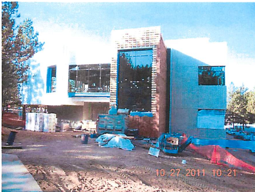
Shingles on East end.
