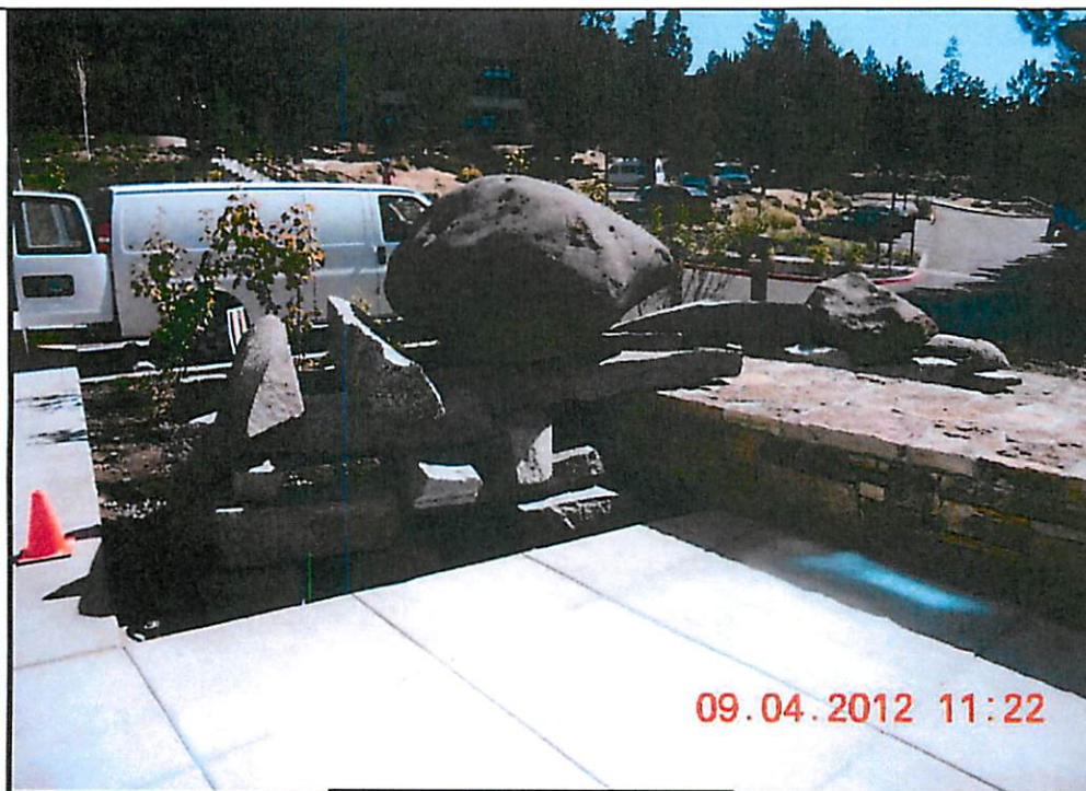
Exterior art in progress
